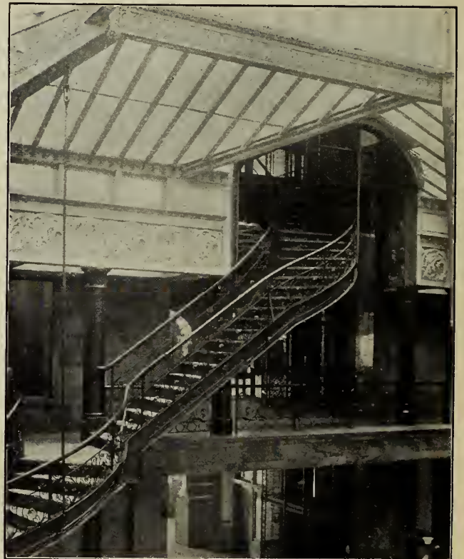
D.—STAIRWAY, MILLS BUILDING, SAN FRANCISCO. Cast Iron Stringers and Risers, Rail Wrought Iron.
